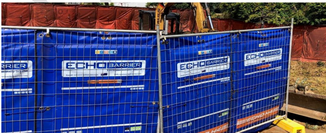
Figure 4 Example of Localised Acoustic Screening (during concrete breaking works)
